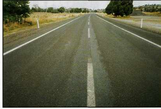
Left: The pavement surface was badly deformed with wheel tracks varying in depth from about 50 mm-100 mm. Right: The finished recycled pavement with a Chipseal.
