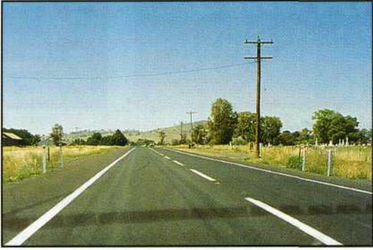
Left: The pavement surface was badly deformed with wheel tracks varying in depth from about 50 mm-100 mm. Right: The finished recycled pavement with a Chipseal.
