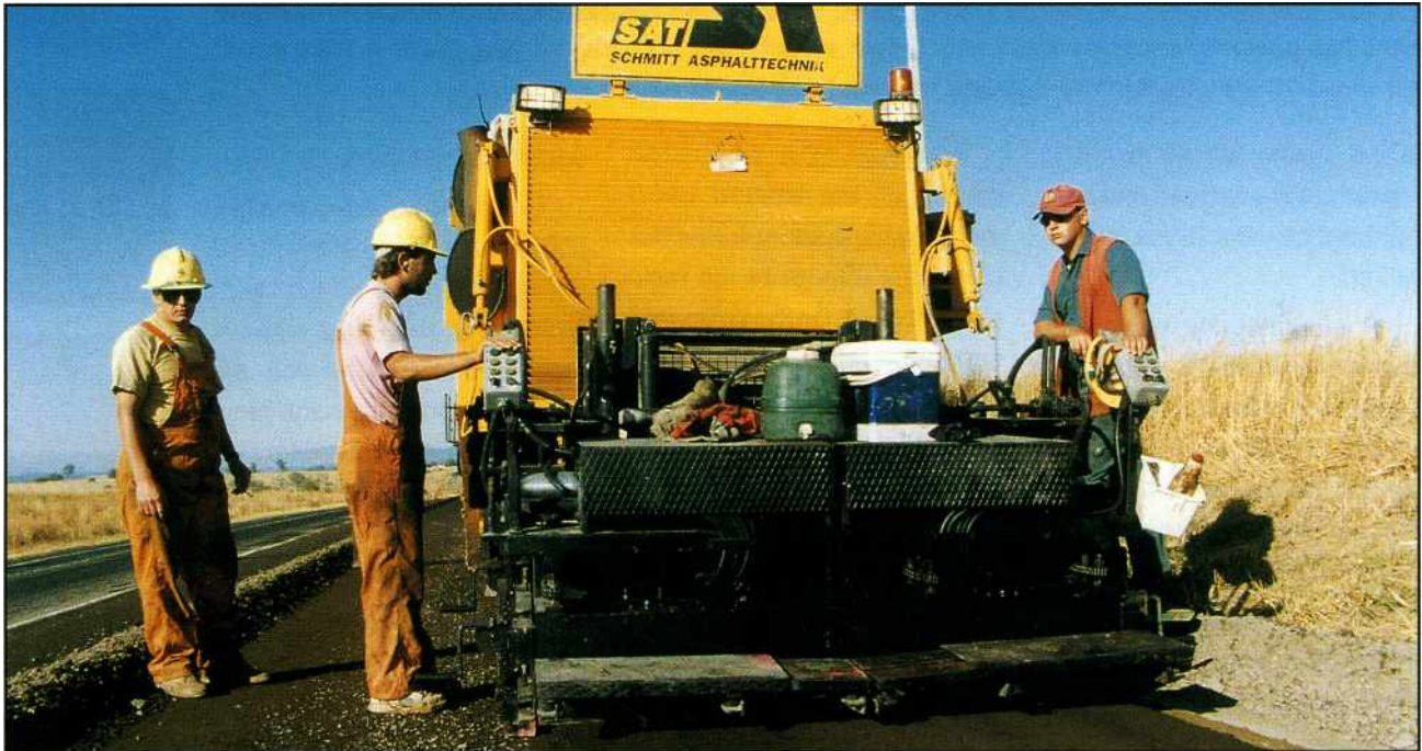
Rear view showing screed and partially compacted surface.
