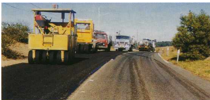
All of the equipment line up and ready to begin another run on Eagleview Road at Campbelltown, where SAMI resealed about 30,000 m 2 of heavily deformed pavement in two days.
