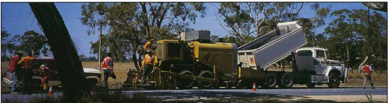
Virgin aggregate being delivered into the hopper of the specialised mixer/paver.
