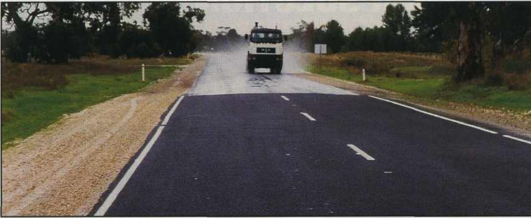
The above shows the improved surface drainage characteristics of a Pave-Flex surface, recently completed by SAMI .
