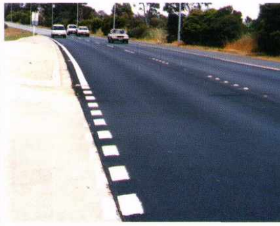
The recycled and restored Freeman's Drive is immediately opened to traffic.
