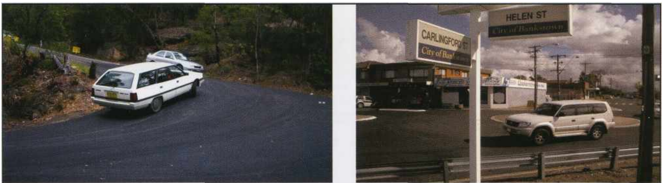
Two examples of roadways under heavy traffic stress and requiring the highest degree of skid resistance provided by SAMI's FricSeal. On the left, one of the many steep hairpin bends on Old Bathurst Road in the Blue Mountains (left) and on the right, one of the busiest roundabouts in Bankstown - both pictured here after SAMI's FricSeal was laid.
