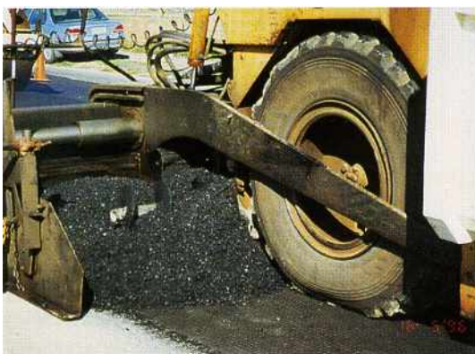
The CompoGrid was placed over a tack coat and did not budge during the paving process.
