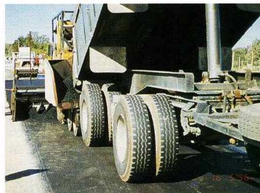
The CompoGrid was placed over a tack coat and did not budge during the paving process.
